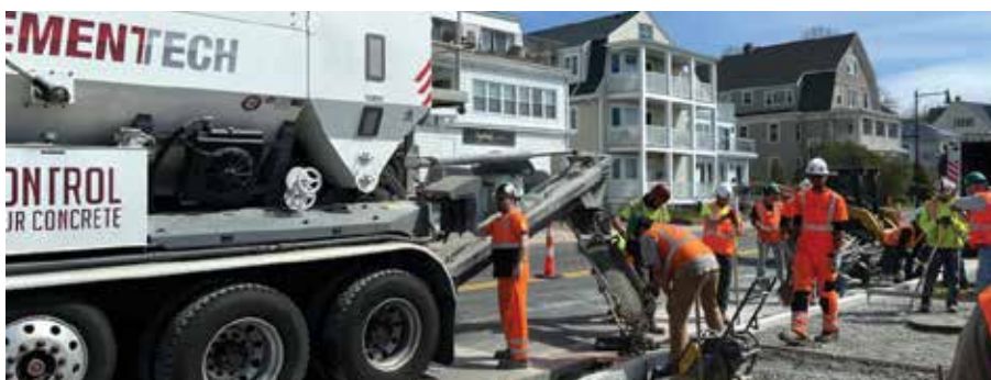
Bus stop construction
